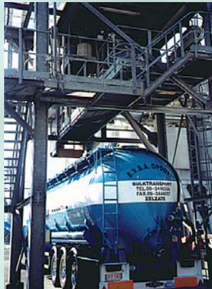
The best location for DeDusting is always at the end of the pellet handling process, before packaging or loading.
